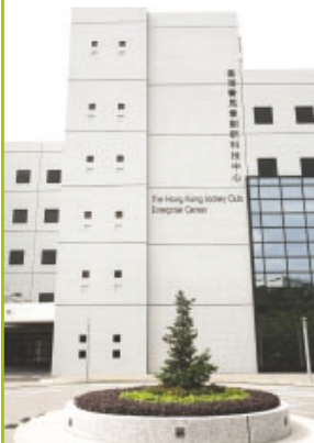
◀ The newest building on campus - The HK Jockey Club Enterprise Center.
